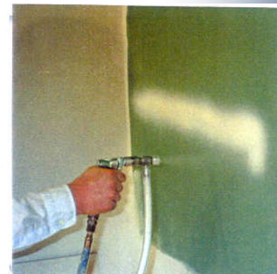
HOLDING THE QUIK GUN 14" FROM THE SURFACE TO BE COATED WILL PRODUCE A 4" TO 5" PATTERN
