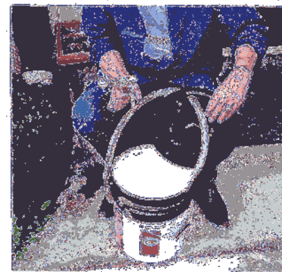
IF YOU MUST STOP SPRAYING EMPTY THE GUN AND HOSE AS INSTRUCTED AND WASH THE GUN THOROUGHLY WITH FRESH WATER.
