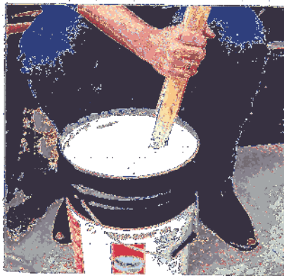
KEEP TEMP-COAT® MIXED AS YOU SPRAY BY STIRRING WITH A FLAT STICK OR PADDLE
