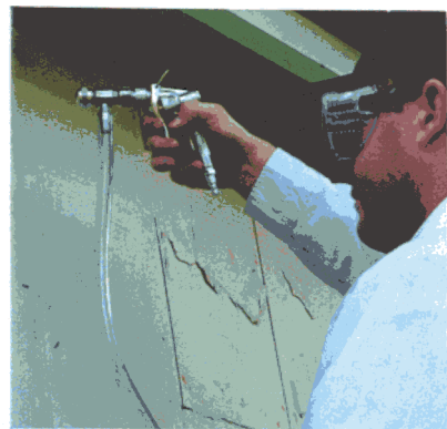
HOLDING GUN CLOSER TO THE SURFACE WILL PRODUCE A SMALLER PATTERN
